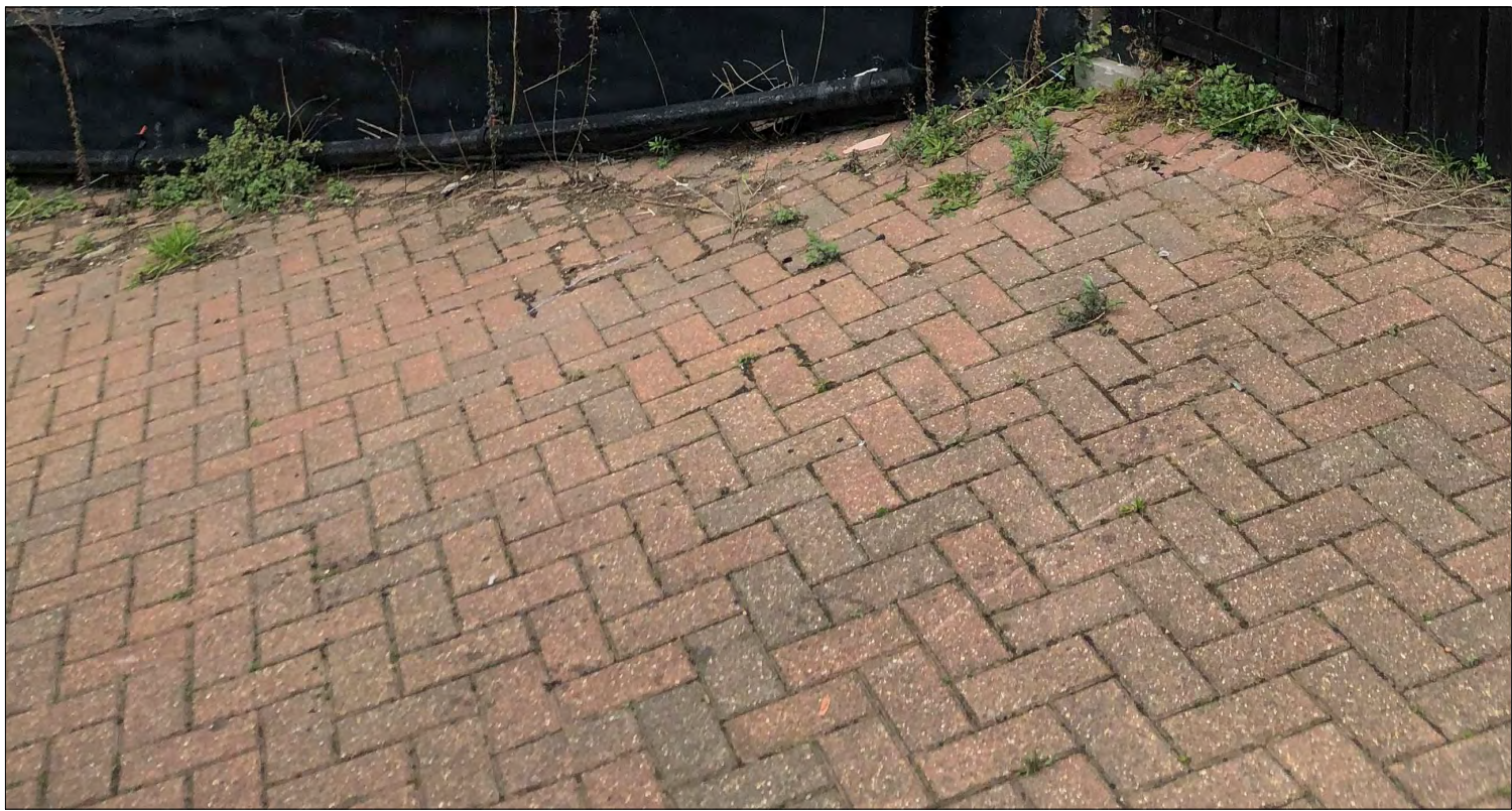
EXISTING HERRINGBONE BLOCK PAVING TO BE CLEANED ANDRE-SEALED
