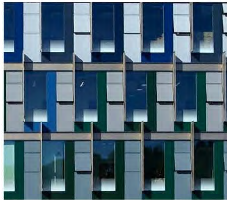
FOR AREAS OF CURTAIN WALLING ALLOW FOR THE FOLLOWING: - 40% FIXED CLEAR GLAZING - 10% OPENING CLEAR GLAZING - 10% COLOURED GLASS - 20% OPAQUE PANELS WITH AN ANODISED ALUMINIUM FINISH - 20% POWDER COATED LOUVRES - PROVIDE A SHUCO CAPLESS SYSTEM - INCLUDE PROJECTING SOLAR SHADING FINS
