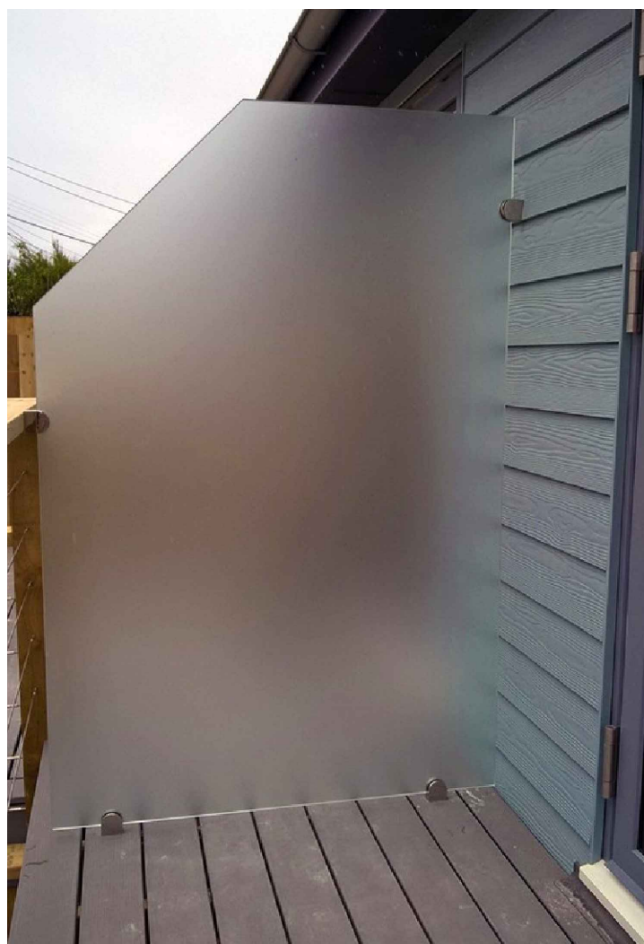
1.8m PRIVACY SCREEN WITH CHAMFERED CORNER
